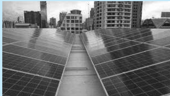
Picture 2 Installation of solar power generation system
